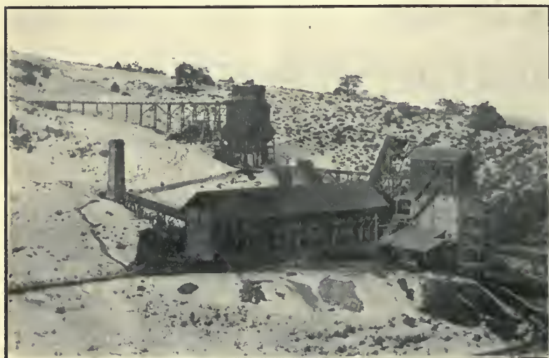
FURNACE OF THE MERCURY MINING CO., IONE, NEVADA.
